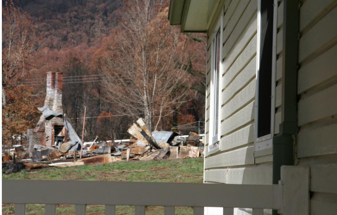
▲ The owner intentionally constructed the house away from vegetation and chose fire-retardant materials, including vinyl weatherboards and uPVC windows.
