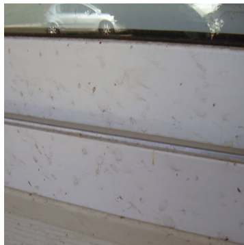
◀ ▶ The vinyl weatherboards and window frames escaped any significant damage and protected the house from ember attack to the interior.
