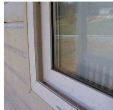
◀ ▶ The vinyl weatherboards and window frames escaped any significant damage and protected the house from ember attack to the interior.
