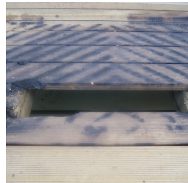
◀ Rowan believes a fire-ball passed across the block along the side of the undefended house closest to nearby trees, dissolving several layers of paint on the timber posts of the rear deck.
