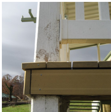
◀ Rowan believes a fire-ball passed across the block along the side of the undefended house closest to nearby trees, dissolving several layers of paint on the timber posts of the rear deck.
